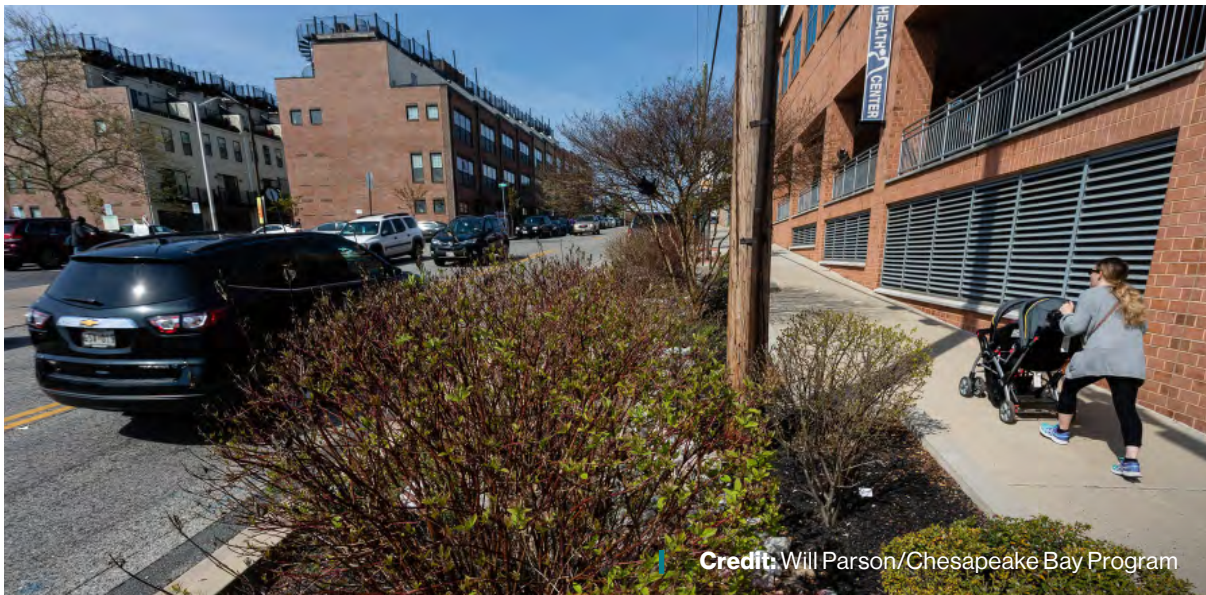
Figure 4. Curb extension on Fleet Street in Baltimore.
