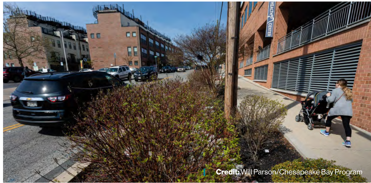
Figure 4. Curb extension on Fleet Street in Baltimore.
