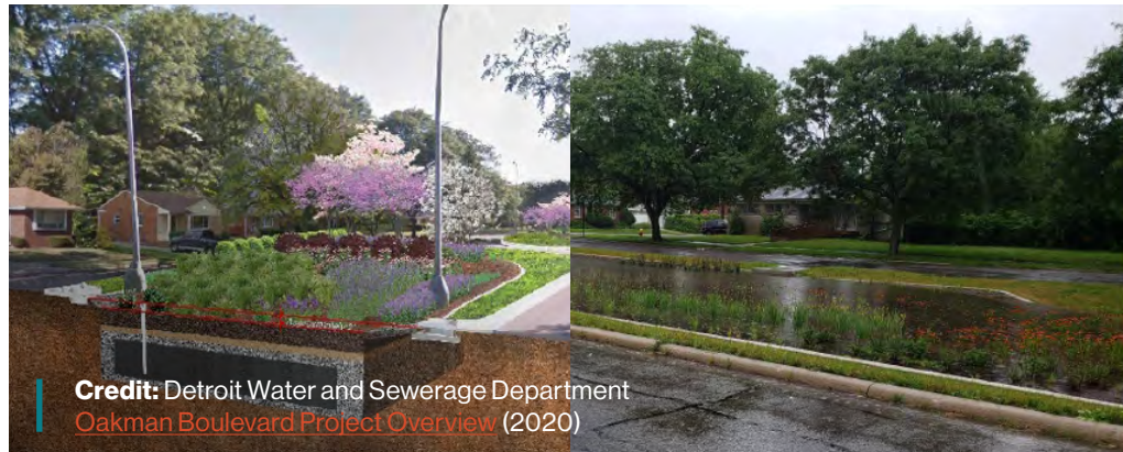
Project rendering cross section (left) and GSI on Oakman Blvd. during 2021 flood (right)
